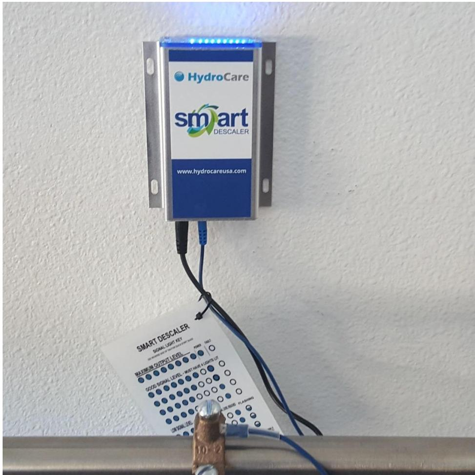
The Smart Descaler™ works with all pipes but must have a metal connection point for signal induction.
